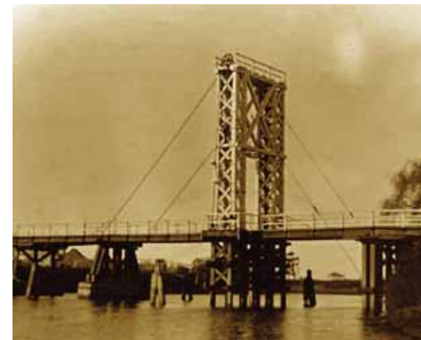
The original Kinchela Bridge.
