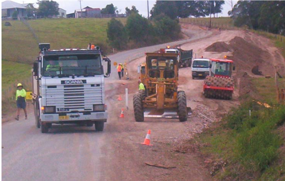
A Shire Services crew at work on improvements to Sherwood Road
