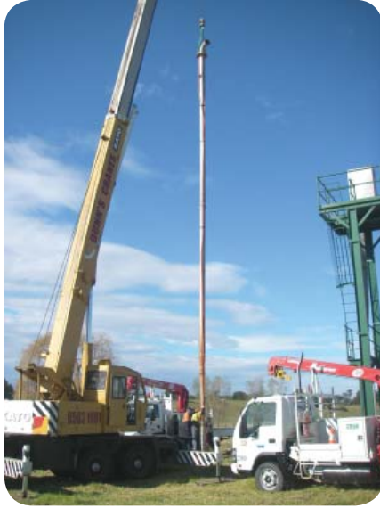
Above: (Left) The bore column is lifted so the pump can be removed and (on the right) Macleay Water staff re-position the pump in the bore hole after the maintenance work is completed.
