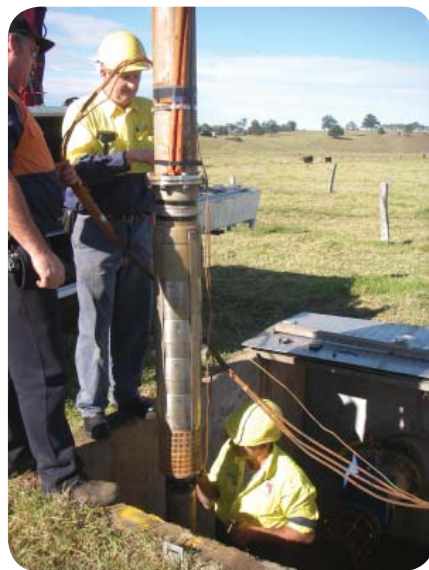
Above: (Left) The bore column is lifted so the pump can be removed and (on the right) Macleay Water staff re-position the pump in the bore hole after the maintenance work is completed.
