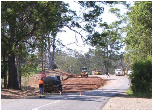
Work in progress at Skillion Flat
