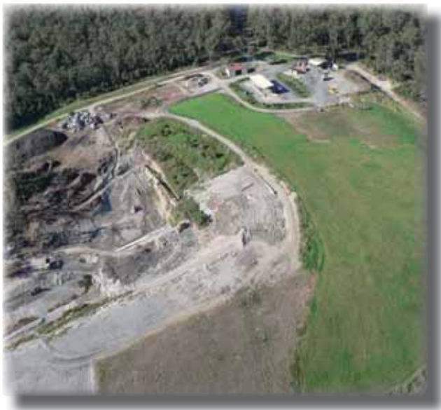
Above: In November 2008 a new Cell was prepared at the Kempsey Waste Disposal and Retrieval Facility on Crescent Head Road.
