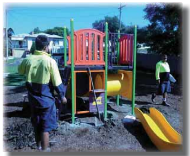
Above: New playground equipment was installed in Flanagan Park, West Kempsey.
