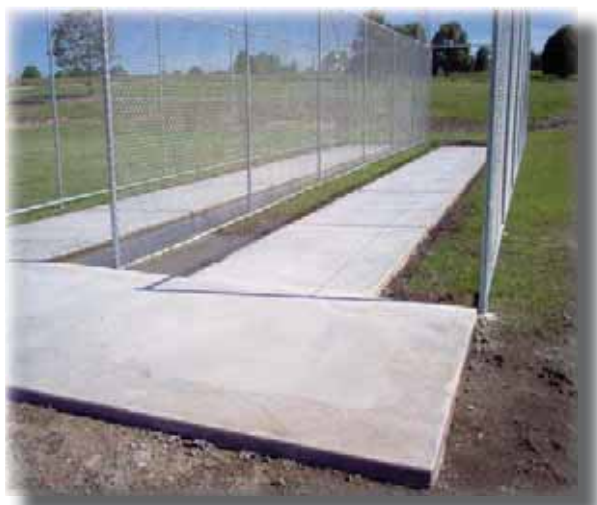
Above: New practice cricket nets were installed at Frederickton sporting fields.
