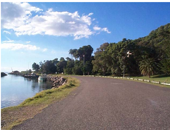
Existing road along SWR Creek
