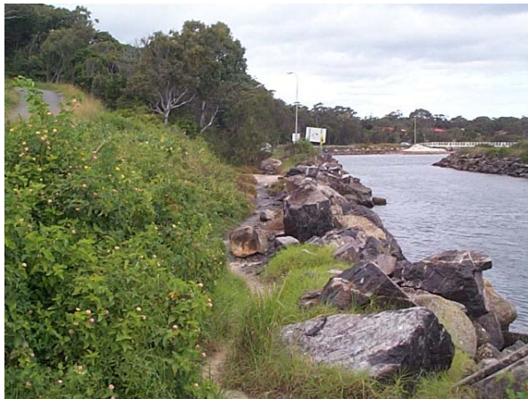
Existing breakwall and track along creek
