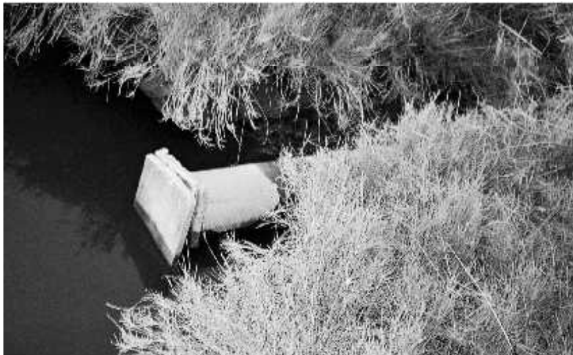
Plate 2: Example of a 150mm pipe with floodgate attached, lying between the open environment and the bermed saltmarsh area.
