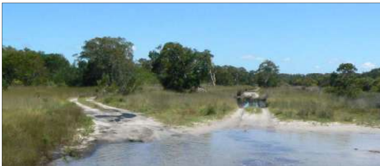
Plate 5 Typical example of disturbance to Saltmarsh communities from vehicles on the southern bank of the creek.
