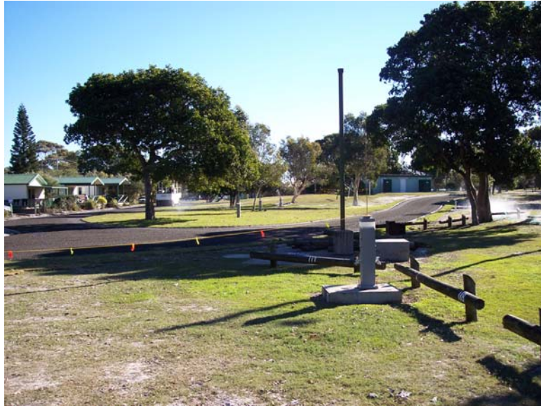
New roadways servicing rear entry to cabins
