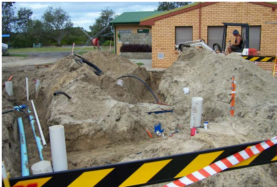
Works undertaken near the amenities block
