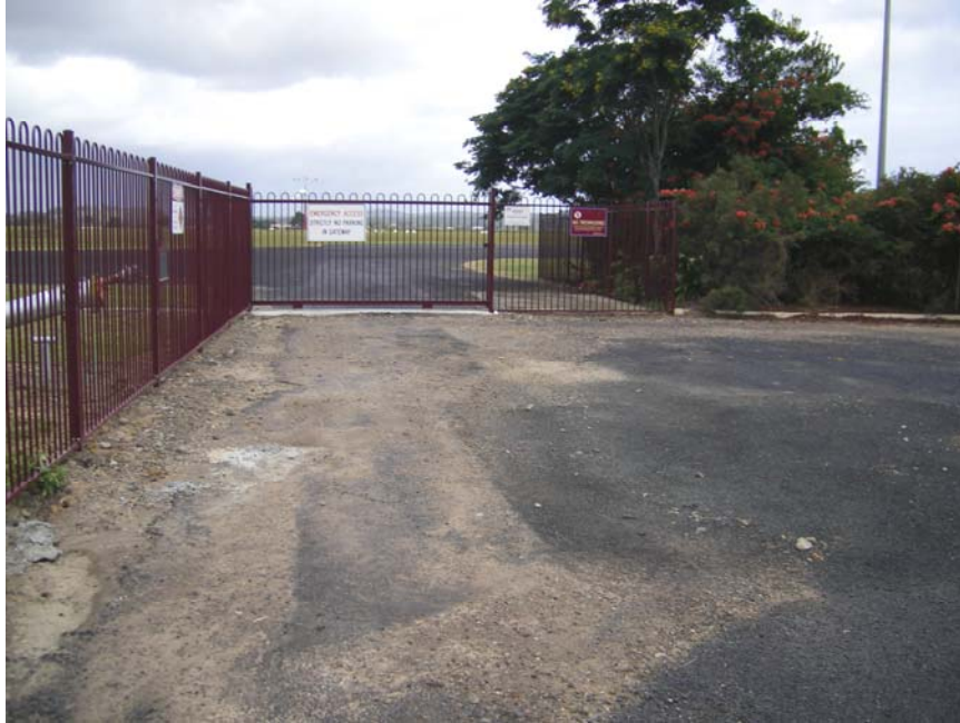
Security airside gate and trenching for security lighting
