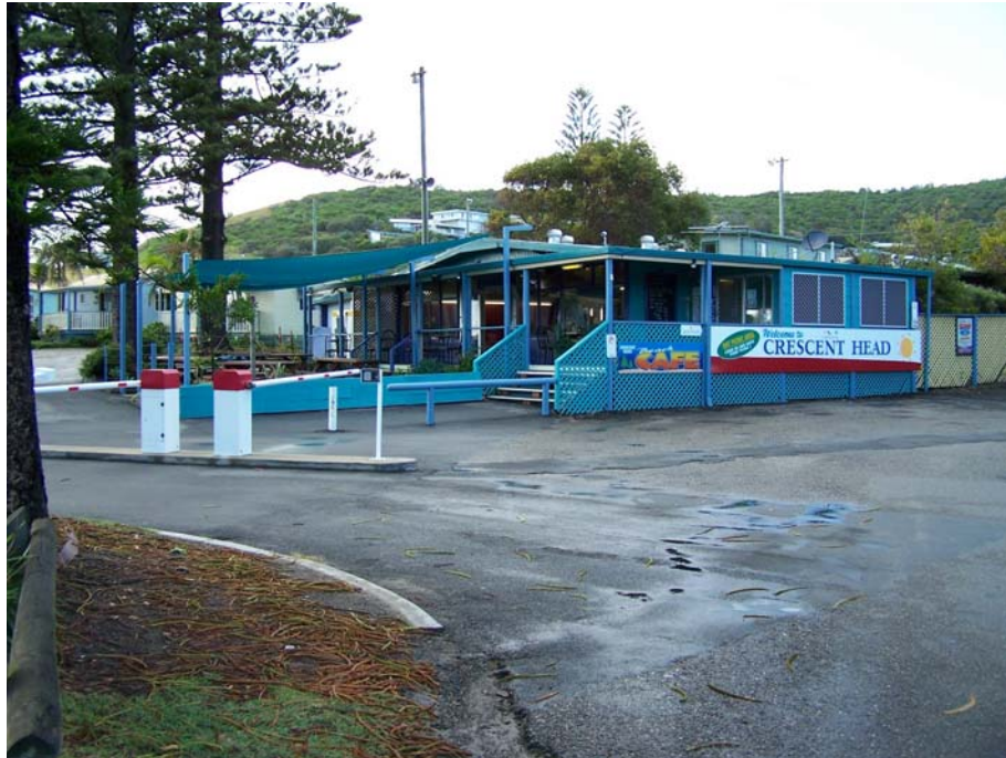
Refurbished Crescent Head Beach Café and Holiday Park reception area
