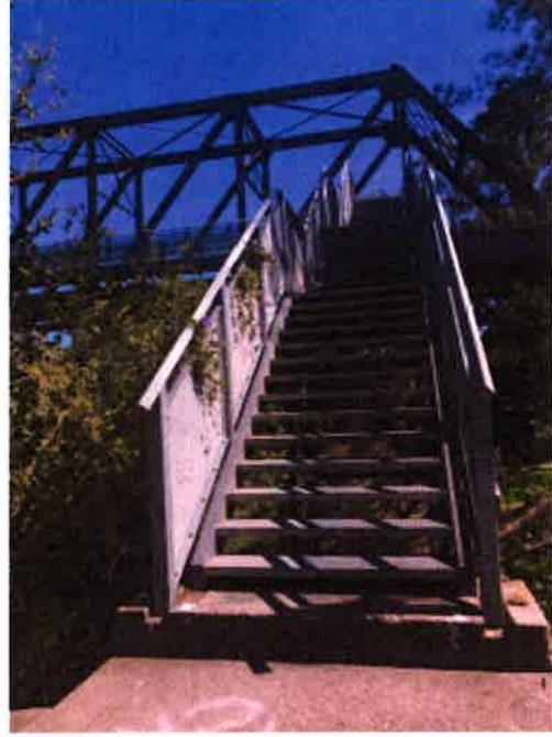
3 flights of 14 steps to pedestrian bridge crossing
