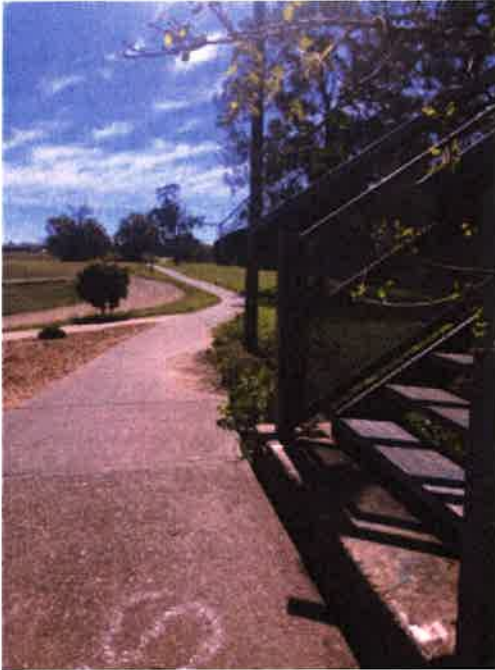
Well-constructed accessible pathway from West Kempsey leading to stairs.
