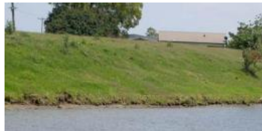
Plate 3.2 Bank Notching by Wind / Boat Waves
