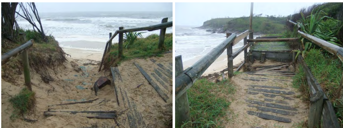
Figure 5-2 Damage to Beach Access and Platform, 1 st March, 2013 (photos: KCC)
