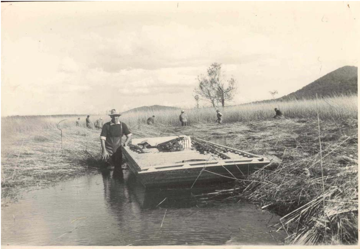
Figure 2-1 Clearing of Belmore Swamp (Source: KSC archives)
