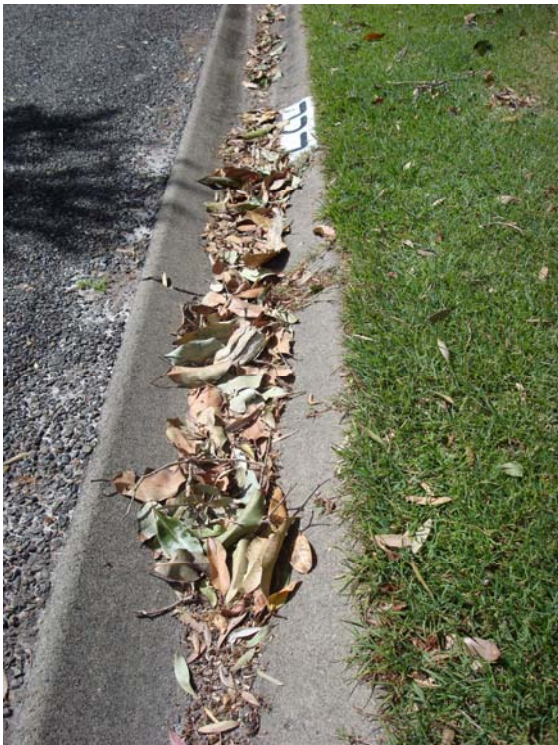
Plate 2.1 Leaf Litter in Caravan Park Drains
