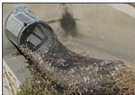
Source: http://www.stormwater.com.au/end_pipe.htm Plate 3.1 End of Pipe Litter Net
