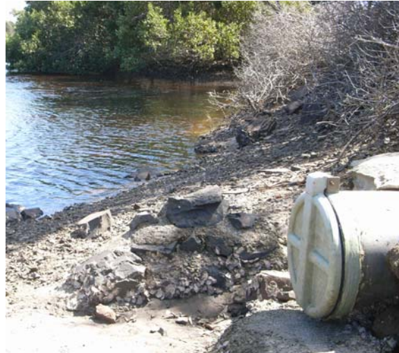
Plate 1.3 Typical Pipe Outlet to Korogoro Creek
