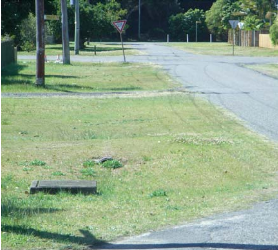
Plate 1.2 Typical Street Grassed Swale in North Hat Head
