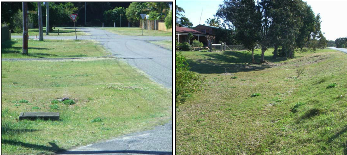
Plates 1-2 Grassed swales and buffer strips have excellent infiltration characteristics and are important in reducing overall pollutant loads in stormwater entering Korogoro Creek (Source: GeoLINK , 2008)
