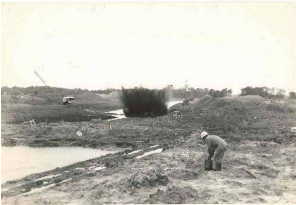
Plate 3 Blasting of coffee rock along Andersons Inlet to create a new drainage channel which eventually would shortcut Clybucca Creek (Source: Kempsey Shire Council archives )
