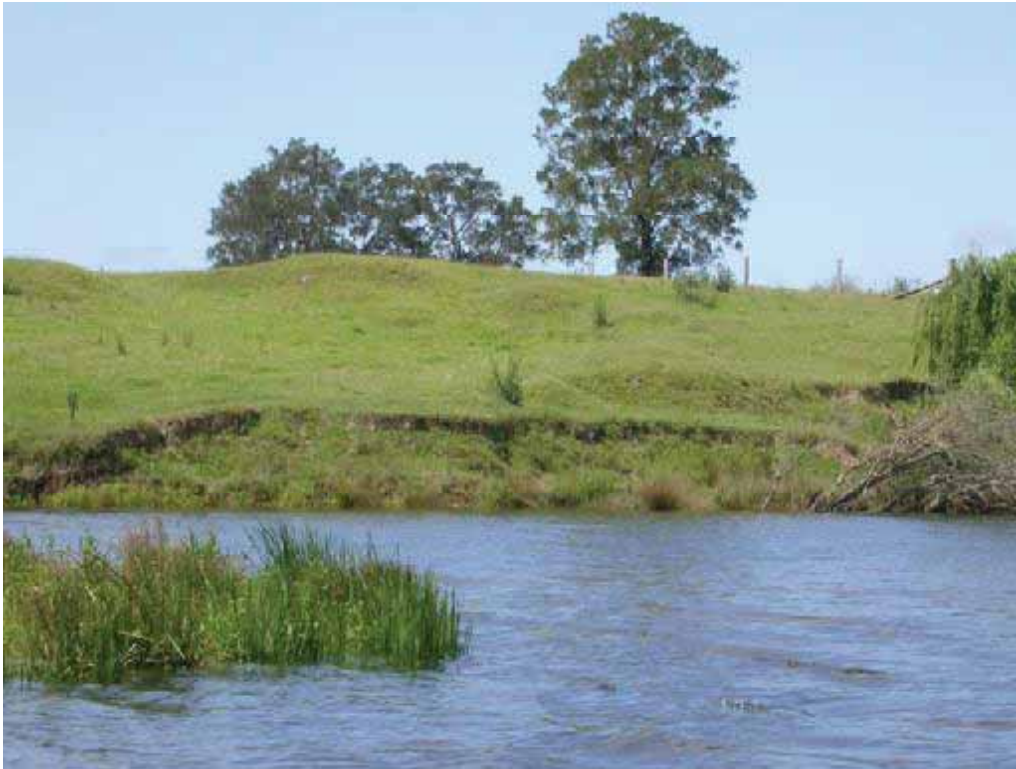
Figure 4 Failure scars (dormant shallow slip) on the toe of the stepped channel margin in Fluvial Reach 1. This stepped bank form is a result of valley confinement and steep gradients producing erosional and depositional units set within the current floodplain.
