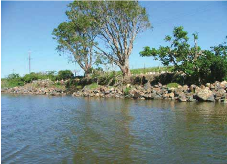
Voluntary Streamcare Grants Scheme Project on the Macleay River . Rock wave barriers, planting and fencing . (E – 0497278, N – 6569866) (ArcView Project # 10 and 14)
