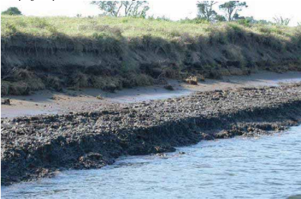
Figure 12 Bank erosion of a ‘deep-water’ profile at Pelican Island – low tide. Note the crab pellets of the basal clays resulting in the basal clay ledge being pre-conditioned to wind/boat wave erosion.
