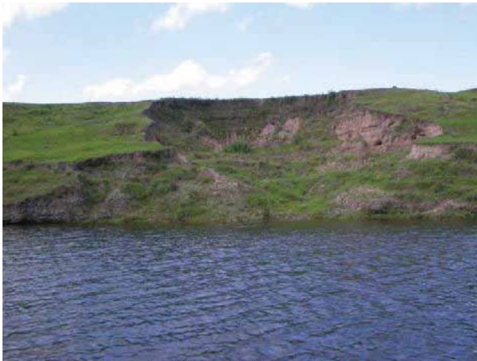
Figure 6 Mass failure (rotational slump) of banks downstream of Belgrave Falls. Bank strength of the Alda Villa and Huntingdon terrace material has been markedly reduced by the replacement of structurally diverse native vegetation with pasture species. Piping and gullying of the slumped zone, along with continued stock access, makes the banks susceptible to ongoing erosion.
