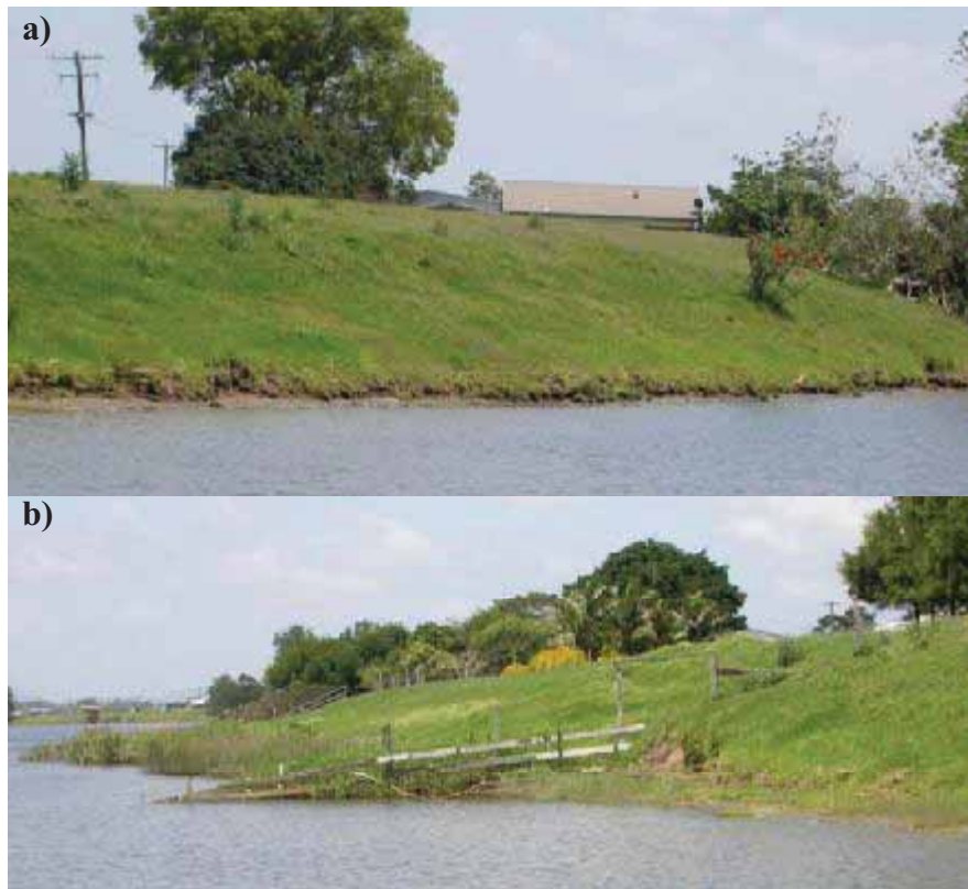
Figure 7 a) Notching of bank toe by wind and/or boat waves in Fluvial Reach 2 b) The impacts of stock on macrophyte growth and toe erosion with varying land use of the channel margin. Property on left has fenced off stock from the channel margin.
