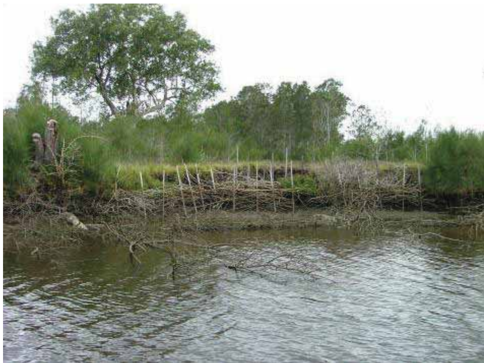
Voluntary Streamcare Grants Scheme Project. Brush groyne erosion control works along the bank of Clybucca Creek. ( E – 0500000 N – 6578100)
