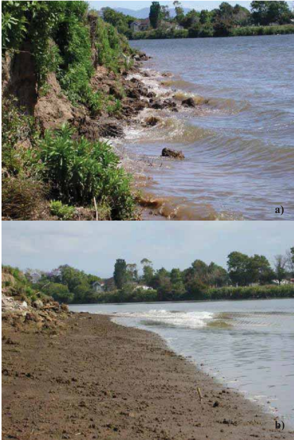
Figure 9 a) Bank erosion on the inside of Kinchela Bend at high tide b) The local hydraulics and basal estuarine clay has resulted in the development of a more subdued sub-water topography with ongoing erosion occurring at mid-high tide only
