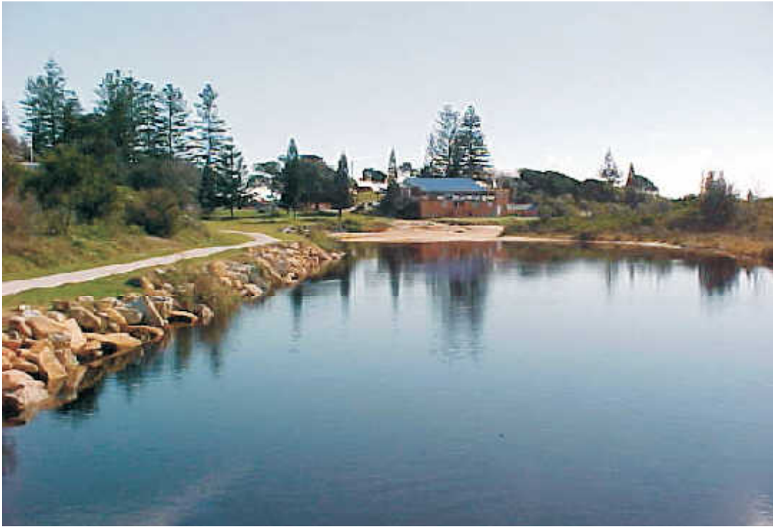
Downstream view from footbridge (18 July 2001)
